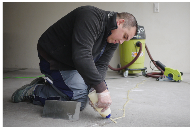
Following the cutting, vacuuming and insertion of the corrugated links, UZIN KR 516 is precisely applied into the joint.
